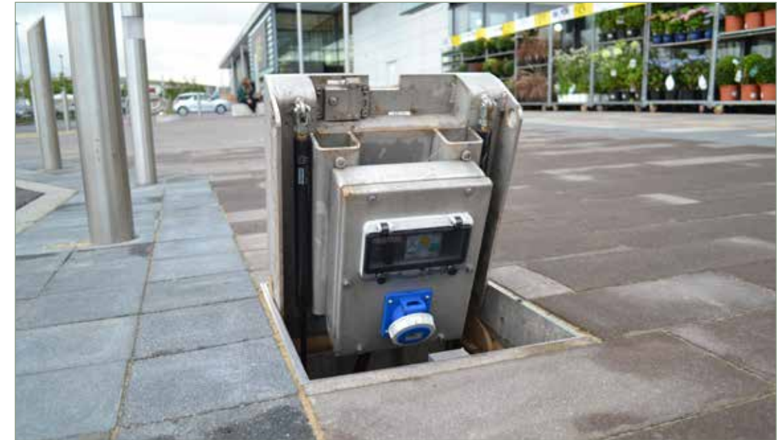
This box is typically used for access by maintenance crews - Power Washers, Lighting, Monolith Displays, Ticket Sales.
